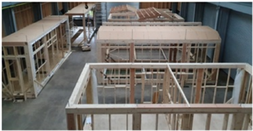
Volumetric housing construction.
